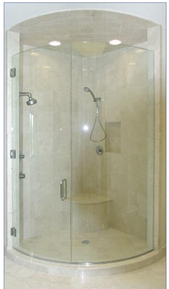
Custom Curved Enclosure
